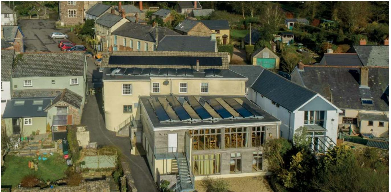
Whilst the optimum location for solar is a south-facing roof, at a 30-degree angle; solar also works well on east-west roofs, with angles between 5 and 40 degrees. The Poltimore Inn is a good example of this, having a 10-degree pitch on a flat roof.
